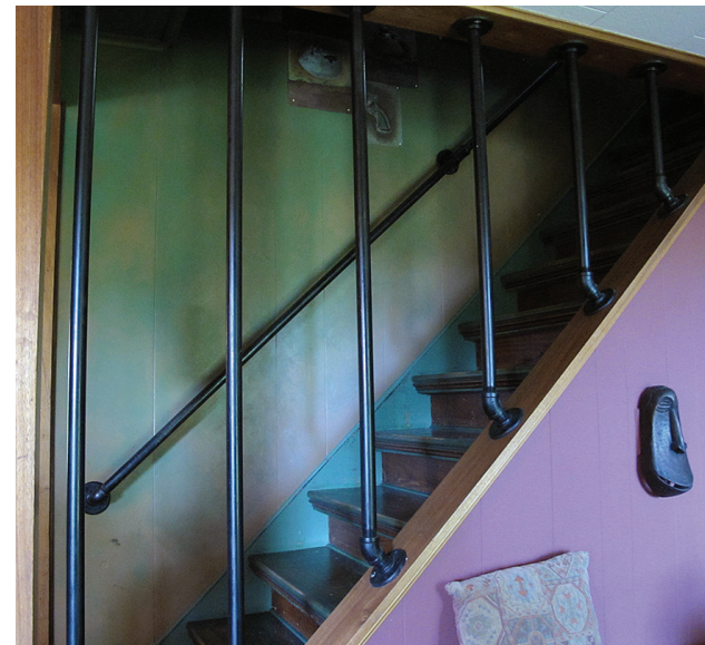
The Drizhal-designed stairway banister is made from black pipe.
