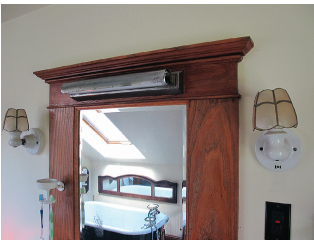
Turn-of-the-century porcelain fixtures with mica shades provide task lighting on each side of this chestnut-trimmed mirror, while a natural spectrum bulb replaces the fluorescent bulb above.
